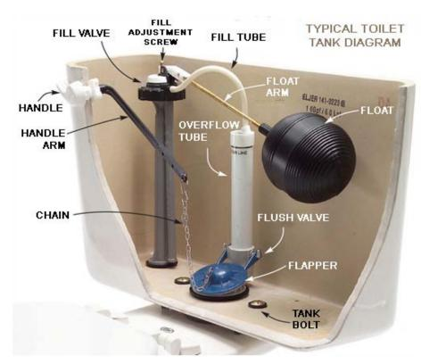
If you see water going out the overflow tube, then the float is probably set wrong, the float has a hole in it, or the fill valve is broken.
